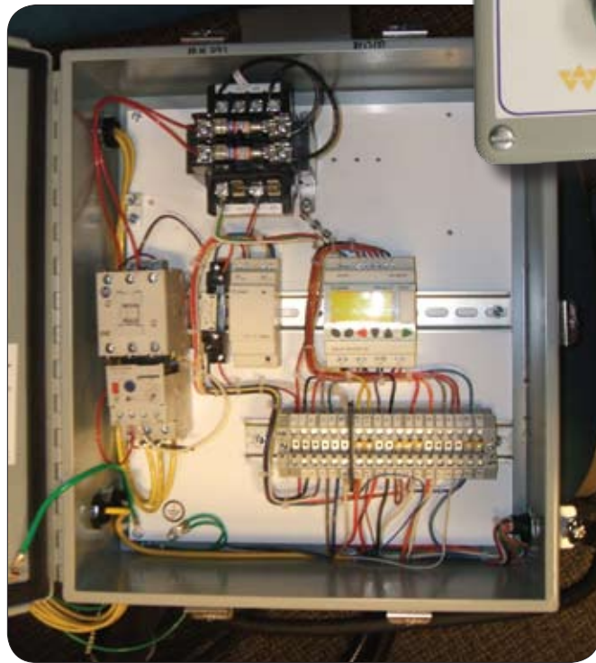
NEMA 4 rated, UL listed control panel
